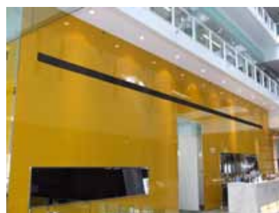
Linear Slot Diffusers in a continuous line
